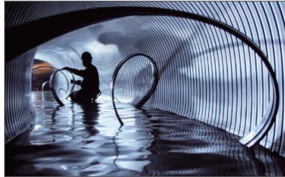
Developed technology (SPR construction method) Photo by Ray Shirao
