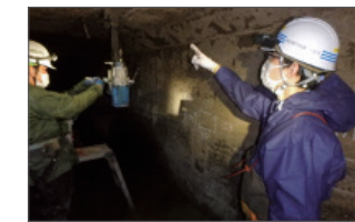
Survey for trunk sewer reconstruction (core sampling survey)
