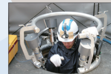
⑨ Hole Air Streamer (bladeless air blower)
