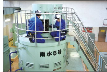
Maintenance inspection work
